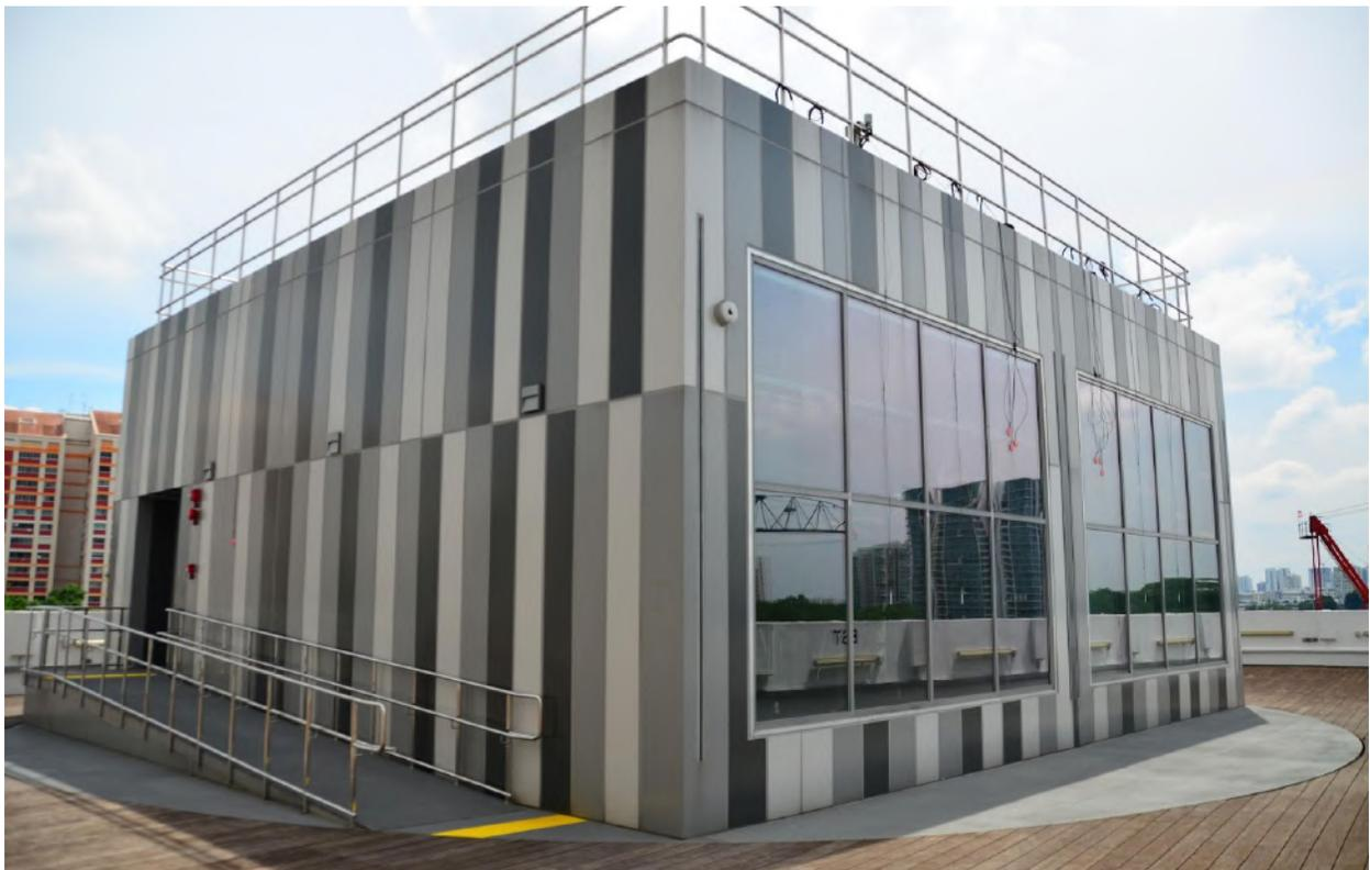
[The BCA SkyLab](#) is the world's first high-rise rotating laboratory developed for tropical climates, modelled after the Lawrence Berkeley National Laboratory's FLEXLAB (Facility for Low Energy Experiments in Buildings). This facility is currently located at the BCA Academy in 200 Braddell Road.
